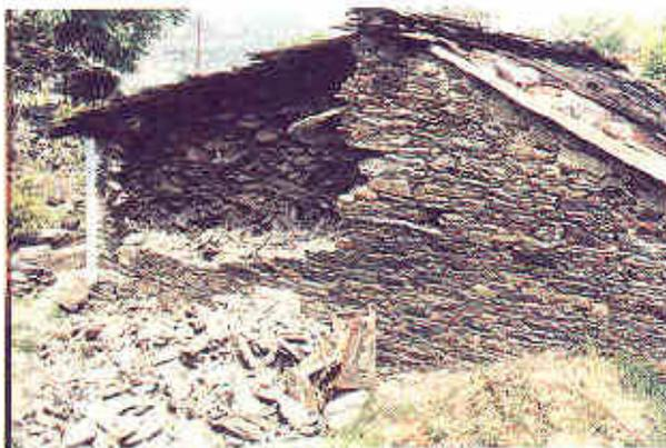
**Figure 7.** Collapse of one of the wythes in a traditional house in slate wafer masonry.
