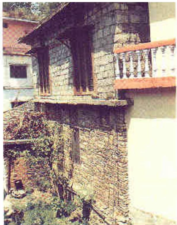
**Figure 8.** Two-storey house at Pipalkoti showing no damage. The ground storey is in slate wafer masonry, upper storey in concrete block masonry has been added later. Both storeys have RC lintel band.
