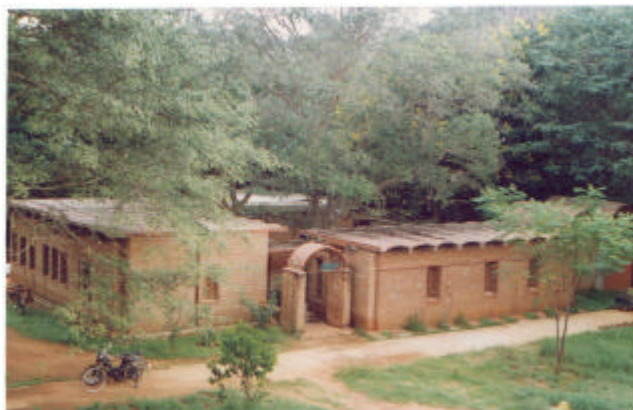
Figure 3. ASTRA office complex (stabilized mud blocks walls and precast beam panel roofs) 1985–86.
