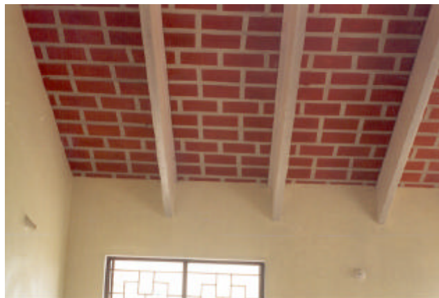
Figure 7. Composite reinforced tile-work panel roof.
