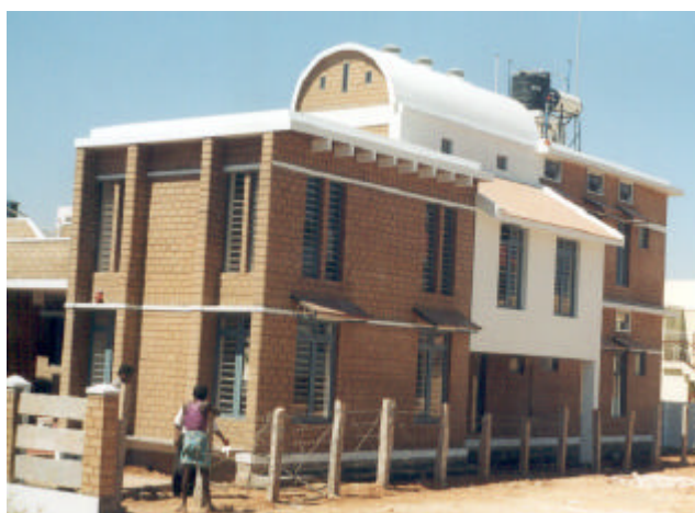
Figure 4. Soil–cement block residential building, Bangalore.
