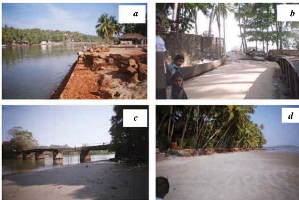
**Figure 5.** Examples of tsunami inundation from northern Kerala. *a*, Collapsed embankment at Choottad, Cannannore; *b*, Country boats thrown inland at Kadalur point, Calicut; *c*, Damaged railway footbridge at Thalassery and *d*, Collapsed laterite banks at Kadalur point, Calicut.
