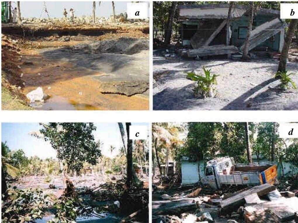
**Figure 3.** Total devastation caused by tsunami at Azhikkal region, south of Kayamkulam inlet. *a*, Deep scouring on the side of the coastal road; *b*, Damaged concrete house; *c*, Totally devastated fishermen colony and *d*, Remains of collapsed houses, including a lorry carried in.
