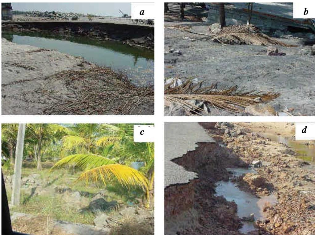
**Figure 4.** Devastation caused by tsunami at Valiazhikkal region, north of Kayamkulam inlet and Edavanakkad, north of Cochin. *a*, Deep trench formed close to the coastal road immediately to the north of Kayamkulam inlet; *b*, Roof of a newly constructed house grounded due to wall collapse; *c*, Boulders of sea walls thrown inland at Edavanakkad and *d*, Deep trench formed close to the coastal road at Edavanakkad.
